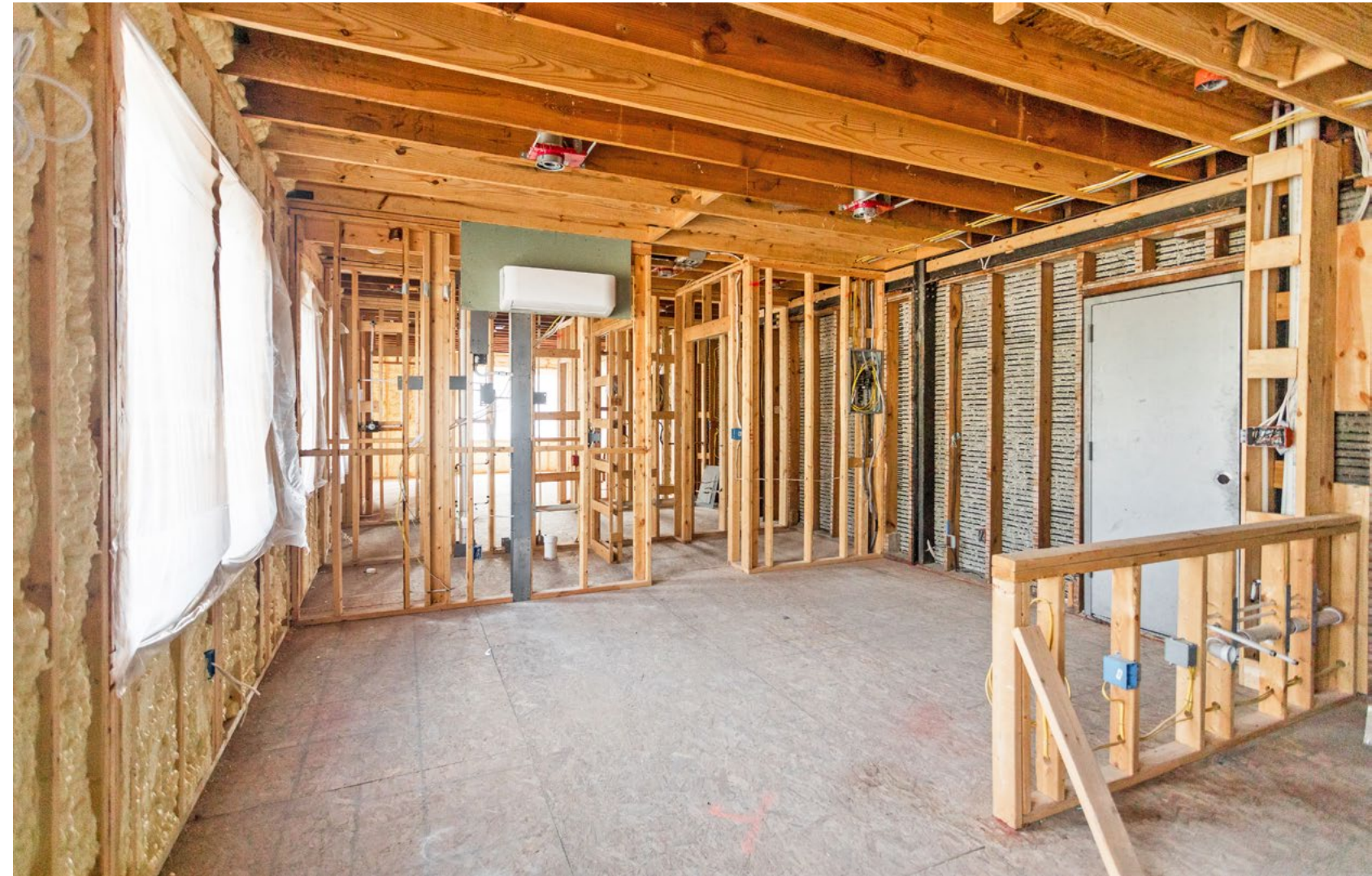
Typical Kitchen & Living Room
