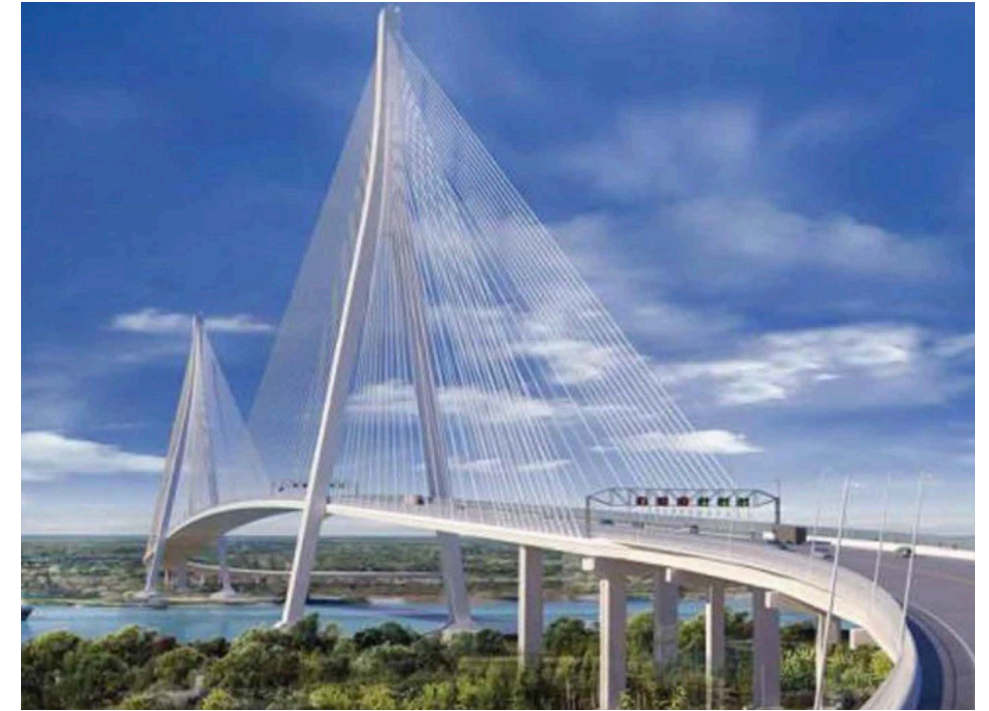
Gordie Howe International Bridge
