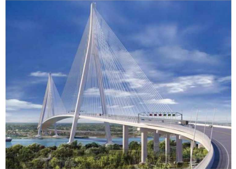
Gordie Howe International Bridge
