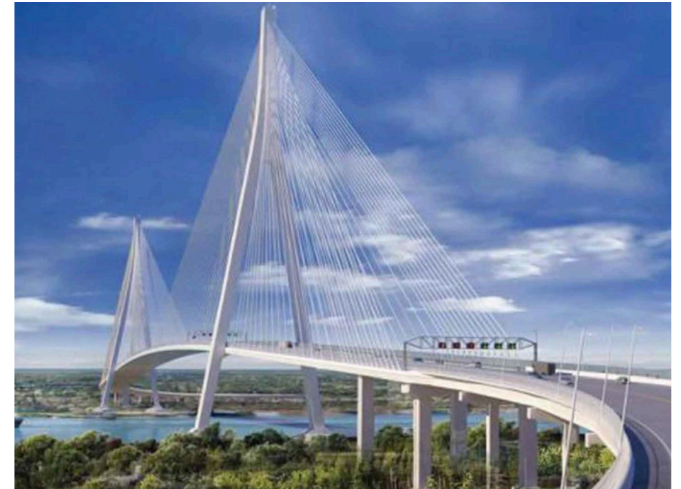
Gordie Howe International Bridge
